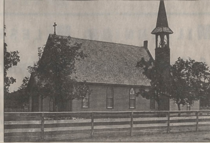
1900s were transferred to this cemetery. (Right) St. John's Episcopal Church, St. Cloud's first church building, was relocated from its original site near the old cemetery. This photo is from 1877.
